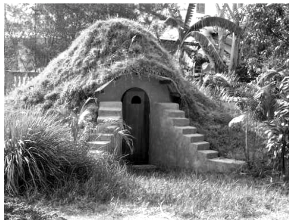
Pic. 5. Example of earth-bag construction
