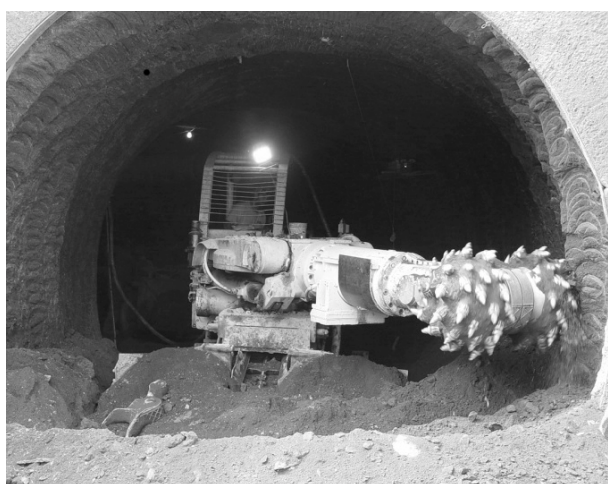
Pic. 3. A roadheader during work procedure
